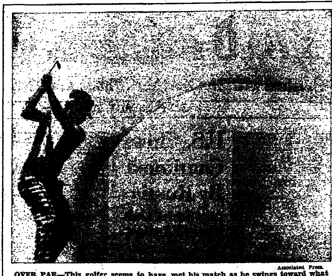
OVER PAR—This golfer seems to have met his match as he swings toward what looks like a giant golf ball. Actually it is an inflatable building, part of the radar installation at a Nike missile site near a Washington motel golf course.
